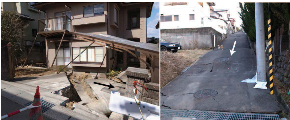
Figure 5. Ground deformation induced by the Midorigaoka #4 landslide in Sendai City. (a) Tension crack at the head. (b) Compressive deformation at the toe.
